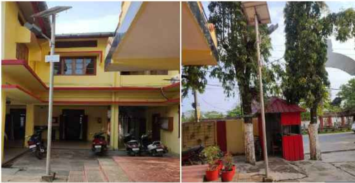
Installation of Solar lights
